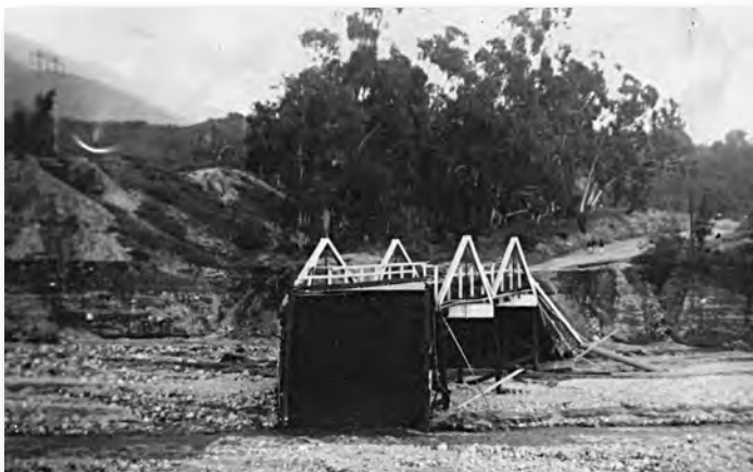
Bridge remains after 1938 flood crashed through Eaton Canyon
