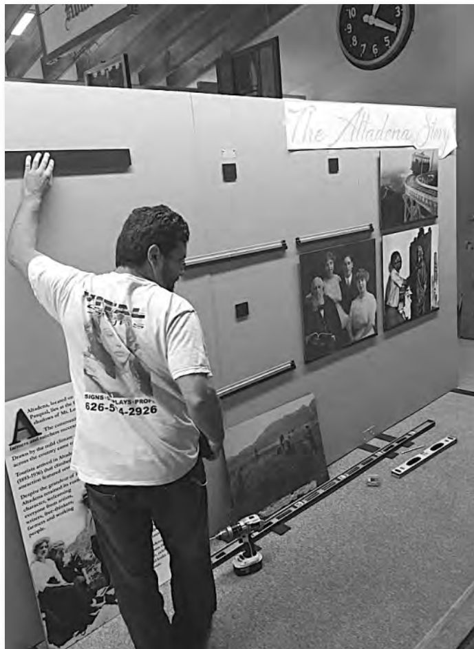
Installation of new exhibit space
